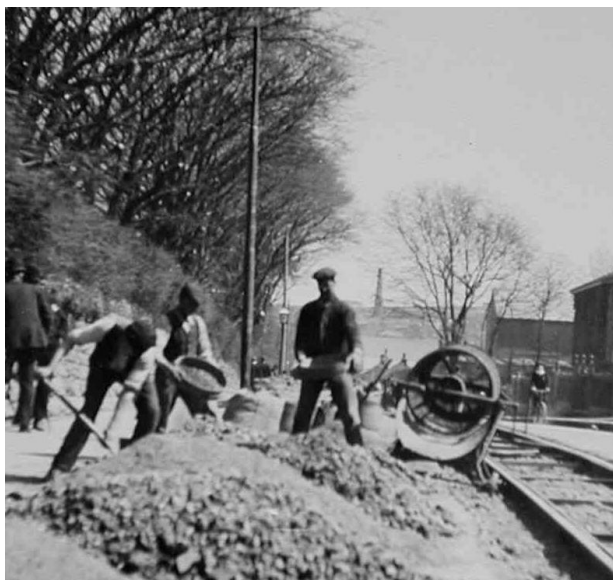
Fig.1 Track Laying in 1901
