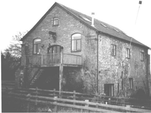
Fig.1 Culm Valley Generating Station at Bradninch (Recent photo by Barrie Phillips)
