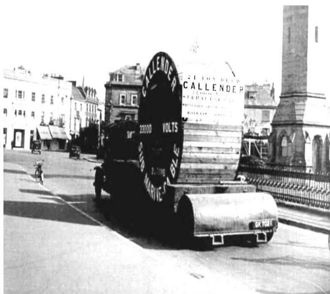
Fig. 5 33kV Cable Drum being delivered for the River Taw crossing in 1934
