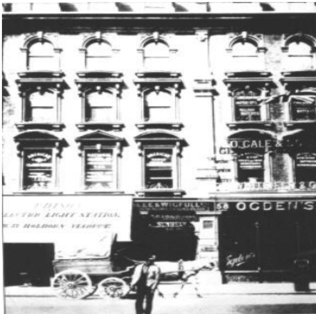
Fig. 1 "Edison Electric Light Station 57 Holborn Viaduct" (words written on the awning)
