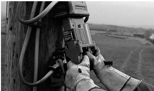
incorporated into a special fuseholder which could be safely closed from a distance after the fuseholder was fully inserted. This would prove if the circuit was still faulty in a safe way. To my surprise they said that they could progress and develop the fuse idea as they were working with a company in Russia, Tavrida, with factories in Moscow and Sevastopol that had the technology to make a small vacuum switch that would fit in the fuse carrier.
