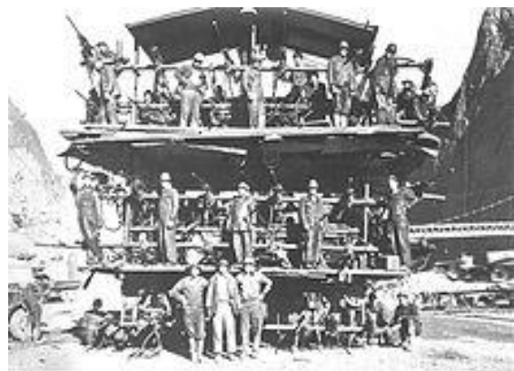
Fig.2 Construction Workers with Jumbo Rig
