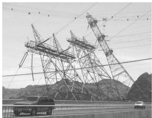
Fig.6 Massive Pylons taking Power away
