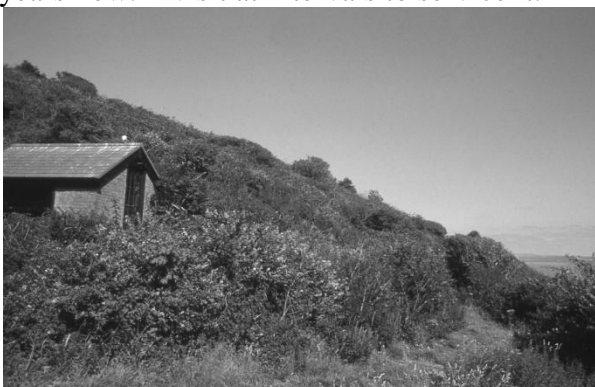
Steep Holm Generator Building
