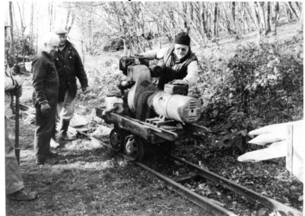
Kelly Mine with Generator on the Trolley
