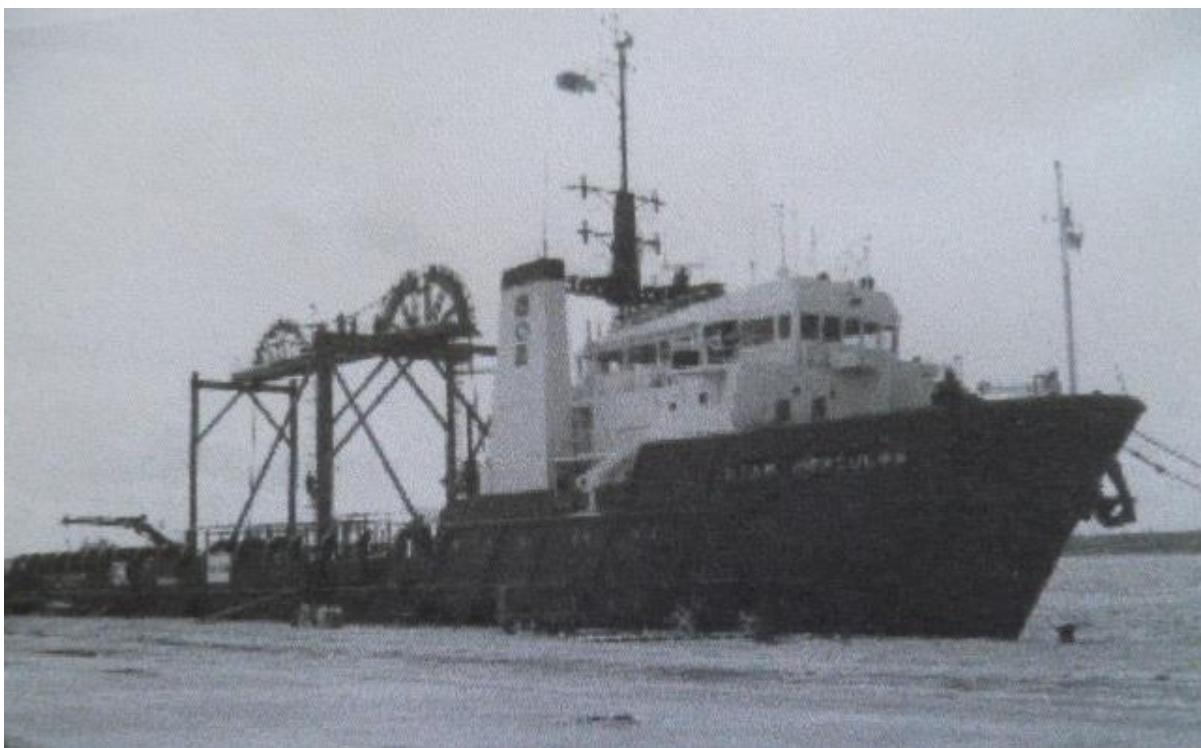
In August 1988 the cable was laid using a converted cargo ship, the ‘Star Hercules’, which steamed at around 1.5 knots from Whitesands Bay to Porthcressa Bay. John Heath from SWEB’s Bristol Head Office was assigned as Project Engineer for the 33kV submarine cable laying, remaining on board throughout the voyage.
