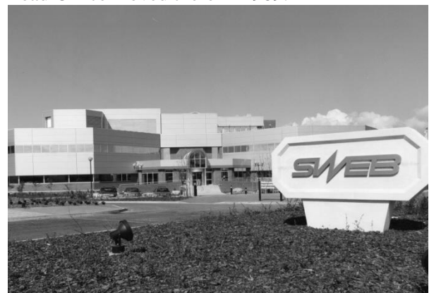
2. SWEB New Offices Aztec West
