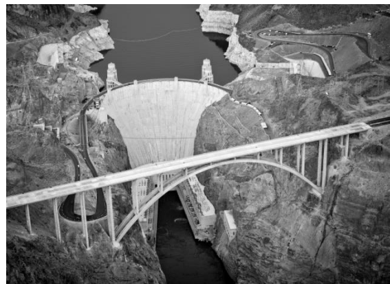
Fig.7 Hoover Dam New Bypass Road
