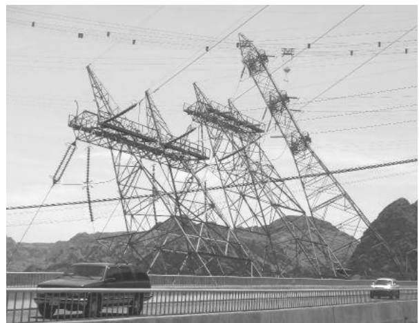
Fig.6 Massive Pylons taking Power away
