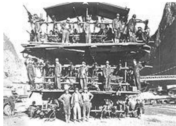
Fig.2 Construction Workers with Jumbo Rig
