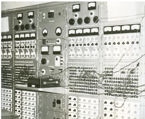
To carry out a network study the first thing to do was to convert all the network constants to per unit values. Per unit values are explained later on. The benefit of using per unit values is that transformer ratios can be neglected. The relevant line and load units are then calibrated and connected to form the network. In the case of load flows, the current and P and Q flows can be measured and tap change positions noted to keep busbar voltages at the required value – 33kV or 11kV.
