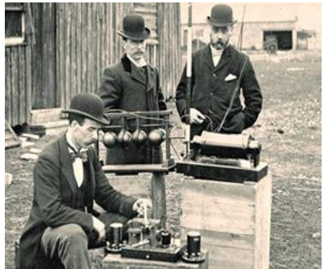
Preece's engineers at Flat Holm
