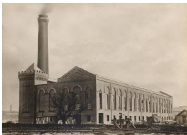
Fig.5 Neasden Power Station
