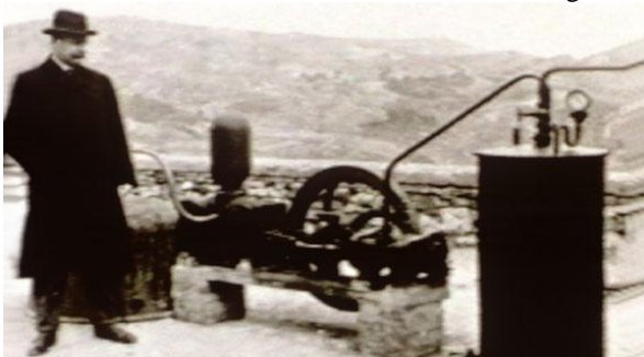
First Geothermal Power Plant, 1904, Larderello, Italy
