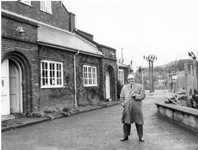
Harry Castle outside Fullbrook Generating Station 1976, then a main substation.
