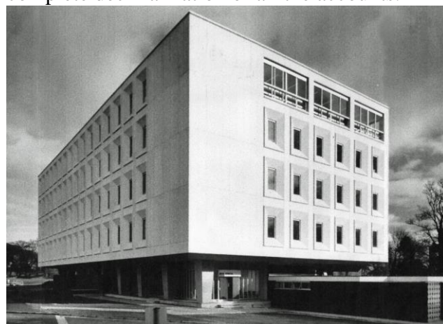
Fig. 6 The Manadon Building in 1971
