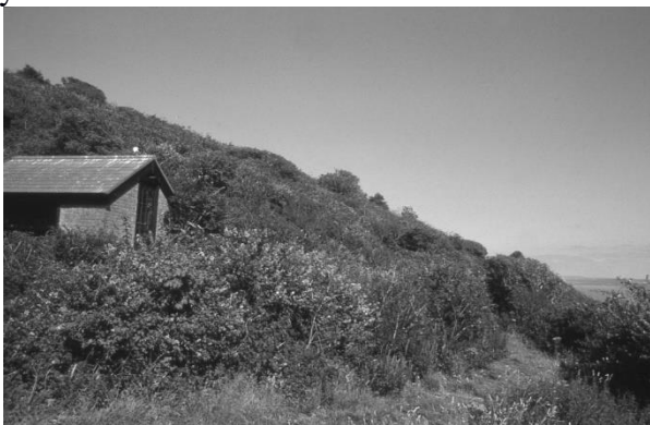
Steep Holm Generator Building
