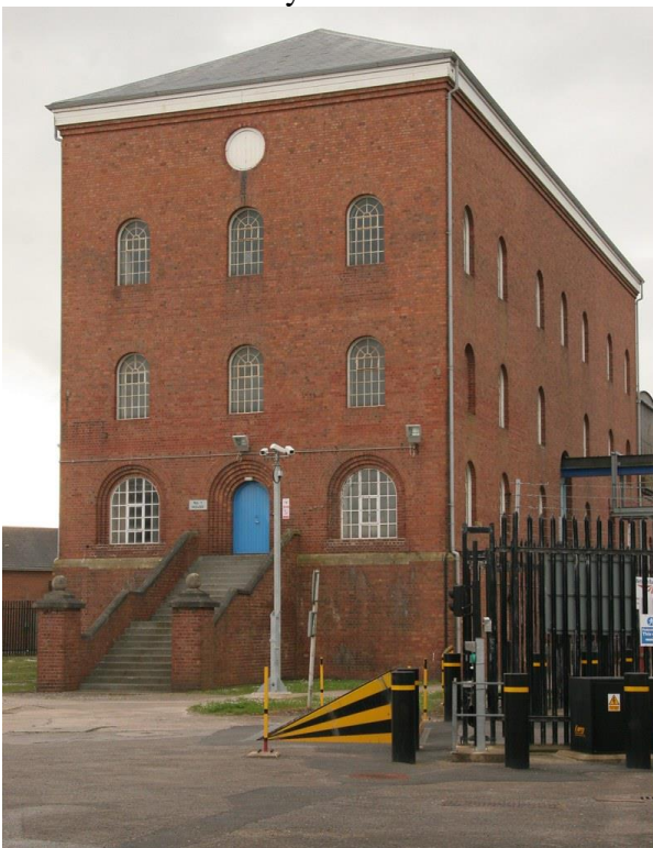
Fig.4 Pumping Station on the Welsh side
