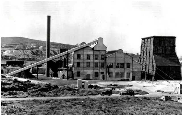
6. ECC Drinnick Power Station
